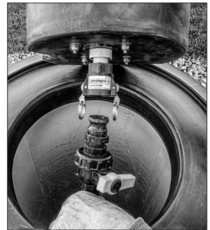
Floatless valve tub disconnected.
